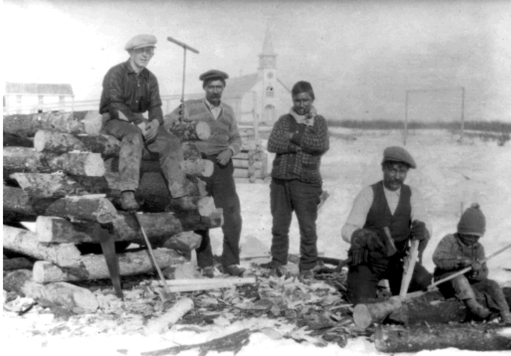
Bridge Construction at Fort Rae.
